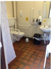
and a shower head adjustable from 1200mm to 1500mm in height. There is a drop-down seat and separate shower chair, and fixed vertical and horizontal grab rails.
