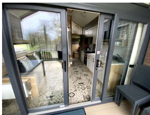
Entrance to the cabin through sliding doors with a 100mm threshold.
